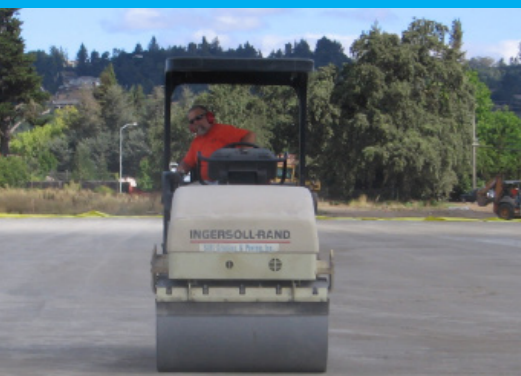
Laser grade and compact to 95% proctor
