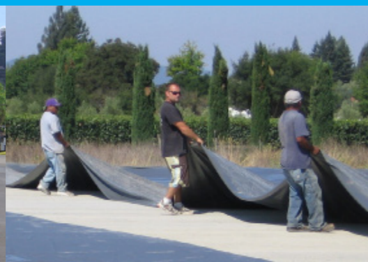
Install non-permeable liner
