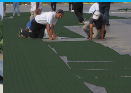
Install tiles across center of field
